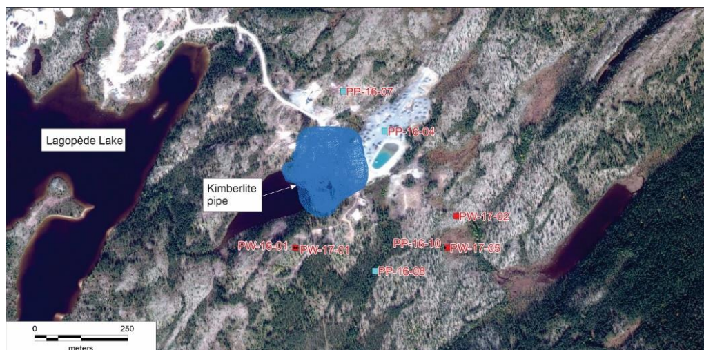
Figure 1: Illustration of the site on an aerial background and representing the kimberlite pipe (blue), the pumping wells (red square), the observation tested boreholes (blue) and the Lagopède Lake.
